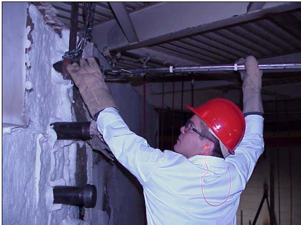
Fig. 12. Inserting particulate testing probe into breaching.
