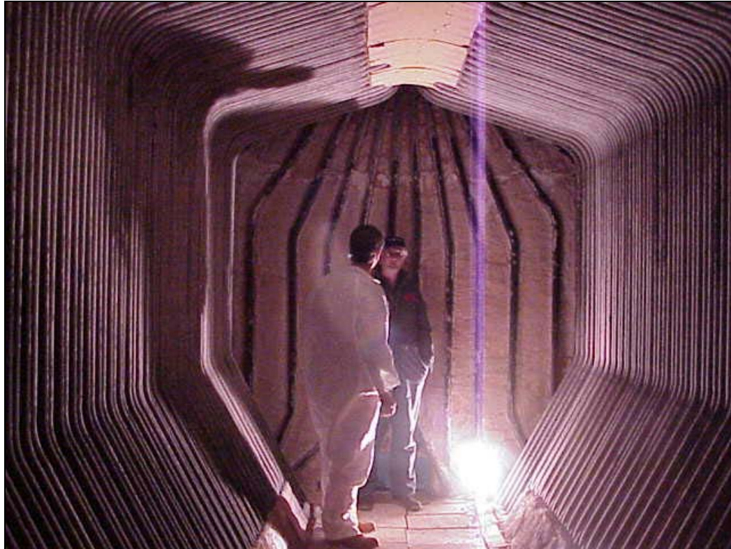
Fig. 11, Inspection of boiler heat transfer surfaces after testing biofuels
